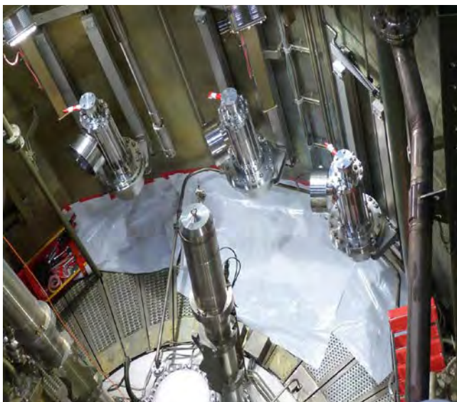
Figure 2: Photo of the three new cooling pumps in the reactor pool of the future ^{99}\text{Mo} -production facility.
